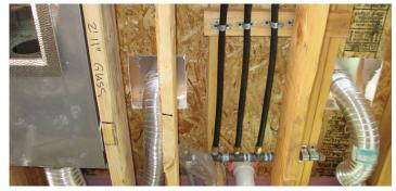
The flexibility and long lengths of CounterStrike® CSST make it perfect for remodel/repair work. It can be pulled like wire, which minimizes the need to remove and replace walls, while at the same time potentially reducing both construction cost and shortening lead times.
