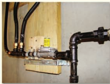
TracPipe® CounterStrike® regulator and manifold station for a 2 psi gas piping system.
